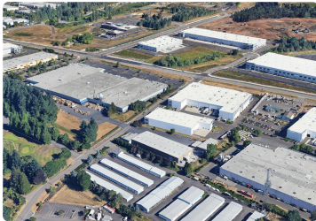
Sherwood Industrial Building SF Leased: 36,000 SF
